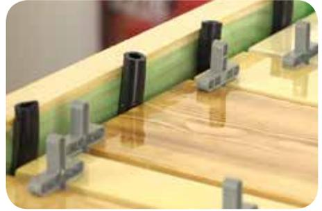
Ideally you need to remove the tile spacers when the resin has started to gel whilst it is still easy to remove them. It can then be left to reach the B-stage again before moving on to stage 3 - the fill layer.
